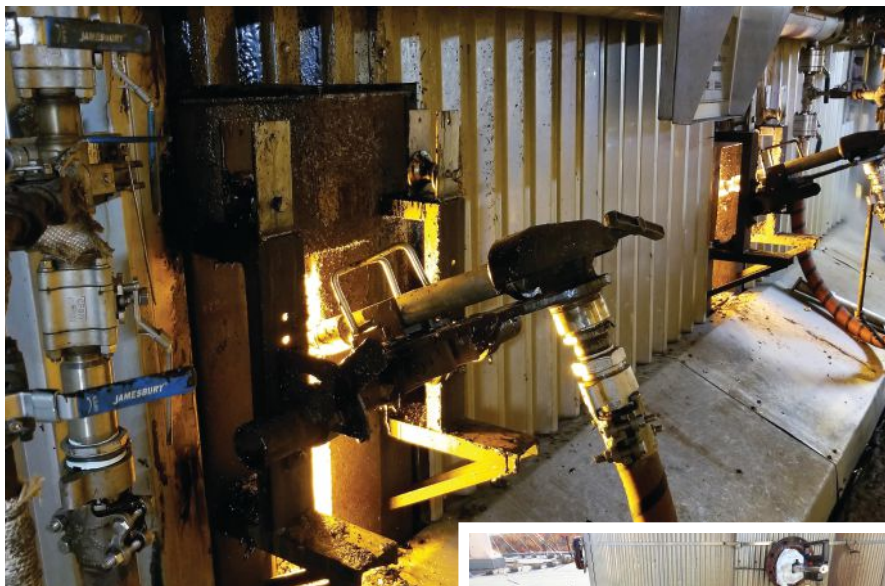
Liquor nozzles on a recovery boiler.
