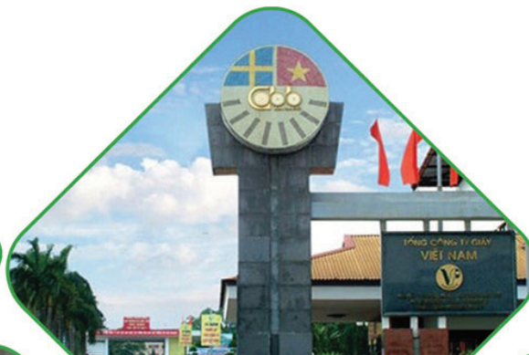
PAPER FACTORY'S SYSTEM OF STORING AND SUPPLYING LIMESTONE POWDER REFURBISHING INVESTMENT VIETNAM PAPER CORPORATION
