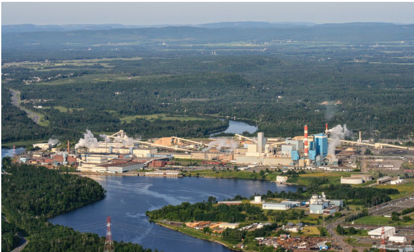
Resolute's Thunder Bay pulp and paper mill, including its bioenergy plant. The mill has a cogeneration facility as well as biomass boilers, three in all, that use waste bark, process residuals and some woodlands residues (hardwood).
