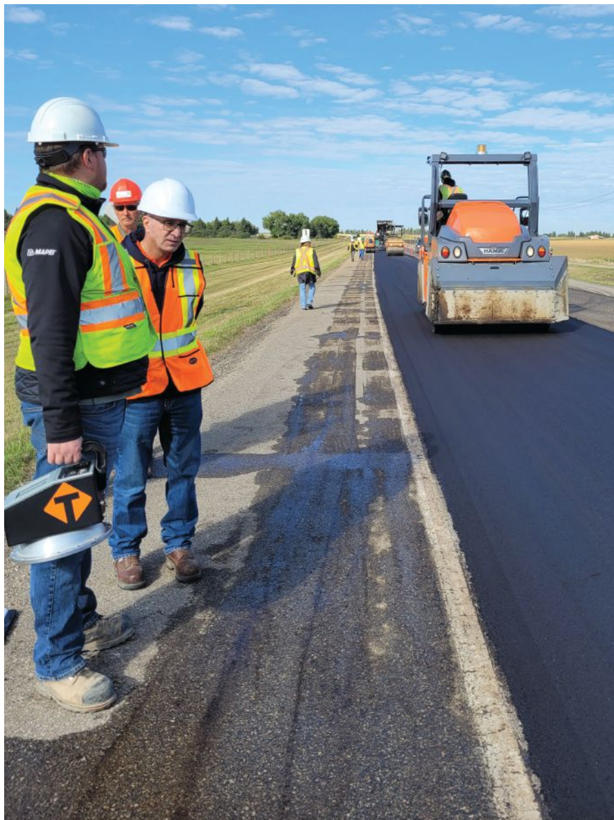
The FPIinnovations research is focussed on finding the right percentage of lignin to substitute bitumen in asphalt mixes without compromising quality.
