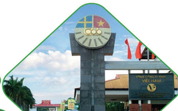
PAPER FACTORY'S SYSTEM OF STORING AND SUPPLYING LIMESTONE POWDER REFURBISHING INVESTMENT VIETNAM PAPER CORPORATION
